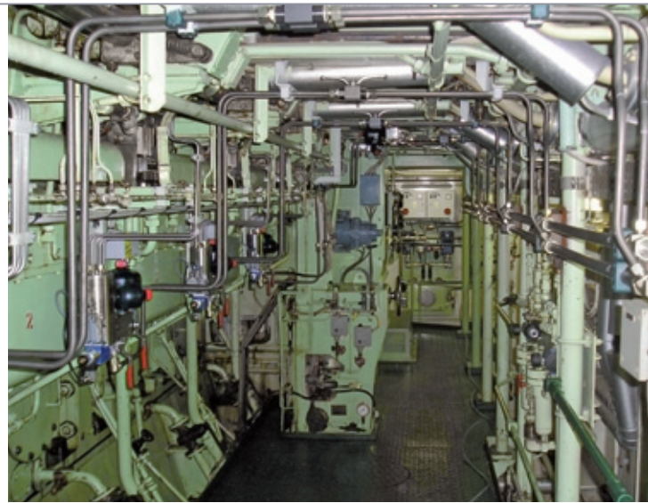
Installation of the Alpha Lubricator
